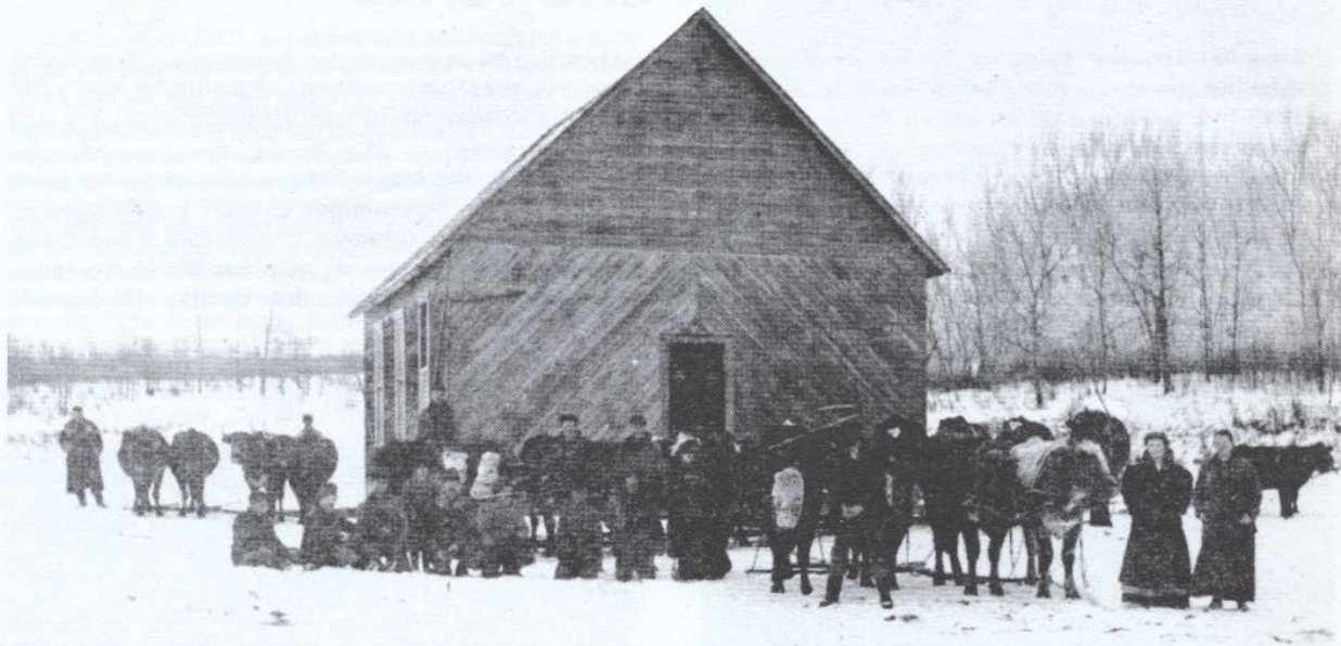
Satersdal Church being moved across the Thief River in the spring of 1908. Ole Listol used twenty-two oxen and received $65.00 for the job.
